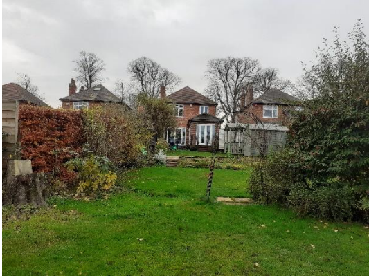
Rear elevation including no's 51 & 47
