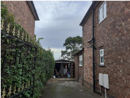
Gap between no. 49 and no. 47
